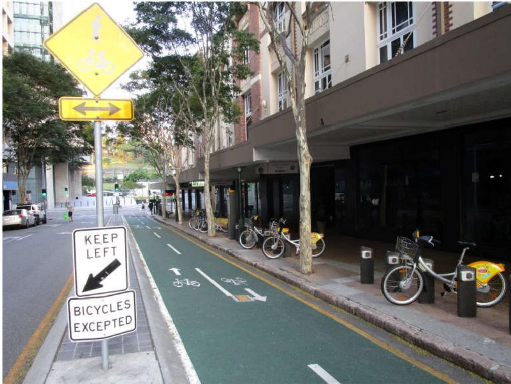
**Image 4:** Tank Street separated bi-directional bikeway. This short section of bikeway connects the Kurilpa Bridge to the law courts and the separated bikeway on George Street. A concrete traffic island separates bikes from motor traffic.
