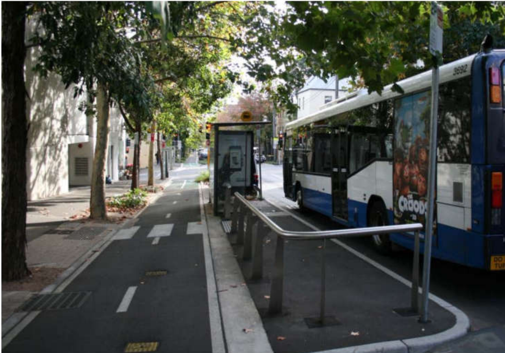
Above: Floating bus stop image from TMR Technical Note 128
